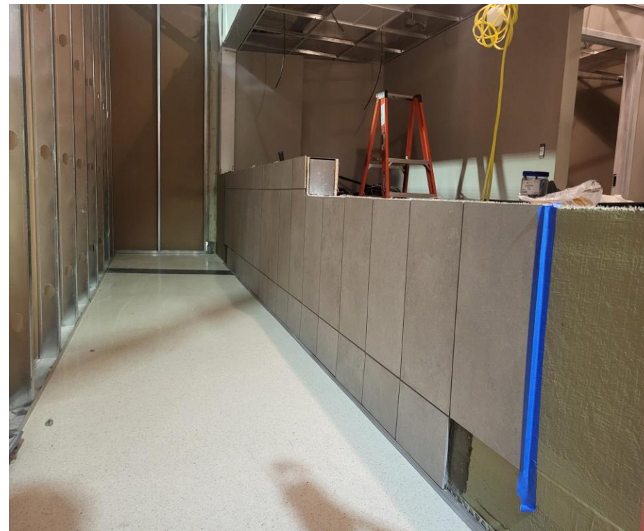
Wall tile installation
